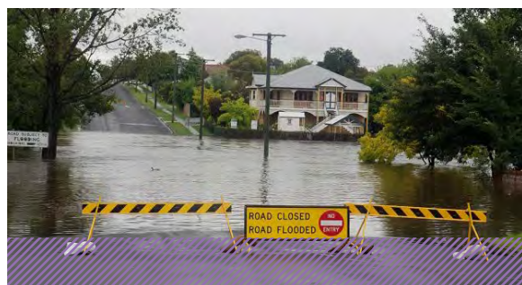
Figure 42: Flooded road on 10 January 2011 in Stanthorpe, Queensland
