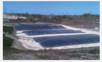
This photo shows three of the biocells at the Swanbank Renewable Energy Facility. Two contain organic waste and one contains leachates (liquid waste); the gas produced from the decay of this matter is collected by the pipes on the left of the photo. Source: Swanbank Renewable Energy Facility
