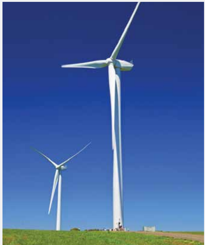
Figure 16. Hepburn Wind Farm 2011.
