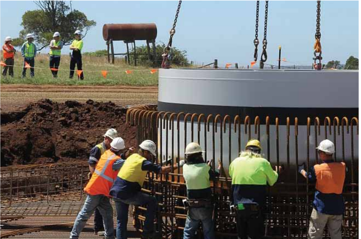
Figure 19. Construction at Hepburn Wind Farm 2011.
